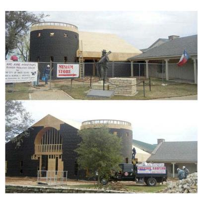
In the photographs above, workers nail wood sheets on top of the rafters as part of the framing of the Research Center roof.
